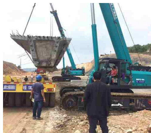
SWTC16在云南省曲靖绕城高速施工 SWTC16 Yunnan province Qujing City Expressway Construction
